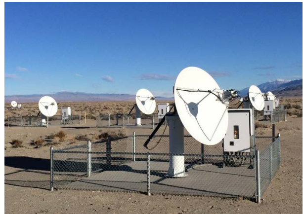
Figure 3: View of six of EOVSA's thirteen 2.1-m antennas.
