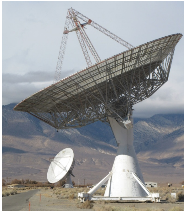
Figure 4: EOVS’s 27-m antennas, used for calibration (and nighttime science).
