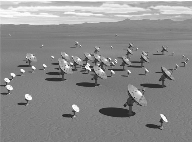
**Fig. 1.**— Artists conception of the FASR array of 2-m and 6-m antennas, in a spiral configuration, as they may appear at a site near the VLA in New Mexico. The LFA elements are not shown.
